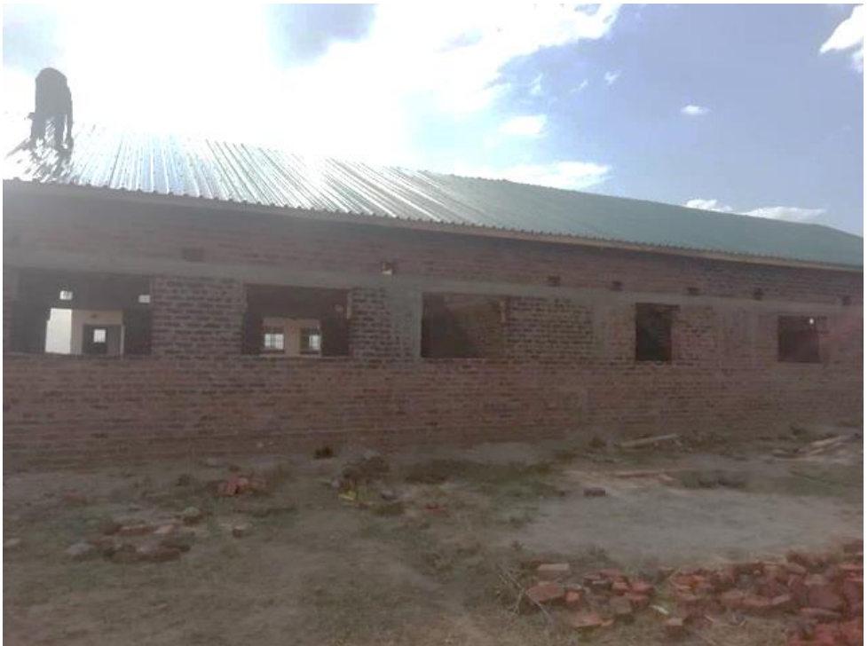
FALCON JUNIOR SCHOOL – ROOF NOW IN PLACE
