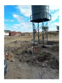
The work involves a site survey (geophysical investigation, pinpoint location); initial drilling (40m) + casing installation; plus further deepening of borehole to 50m+.
